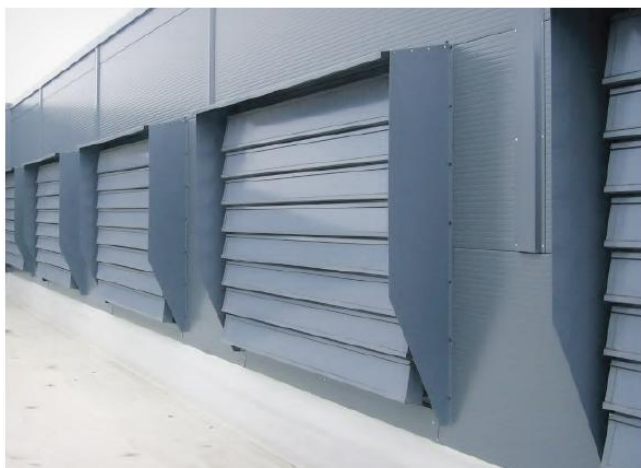
Photo. I-II Vent blades made of aluminum profiles filled with polycarbonate
